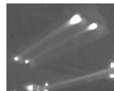
Electrical Hot Spots
