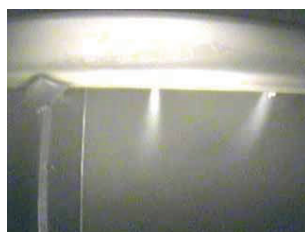
SCR Exit—SBS Injectors Inspection
