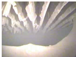
Economizer— Sonic Horn Cavity
