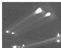
Electrical Hot Spots
